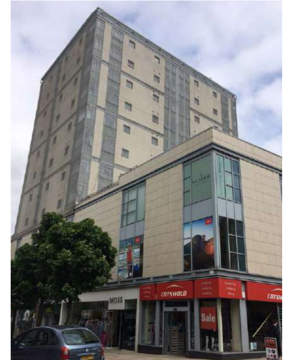
8. Taller buildings within the within the city centre.
