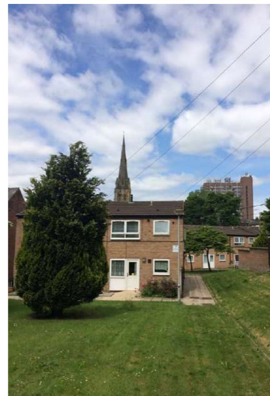
6. View from Avenham Lane with vista to the church spire. 2 storey housing .
