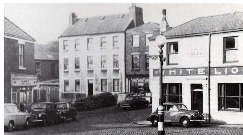
Arkwright House viewed from the south with the now demolished White Lion public house in the foreground
