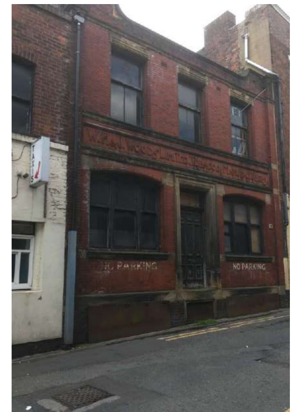
8. Streets with buildings with high quality and historic façades.
